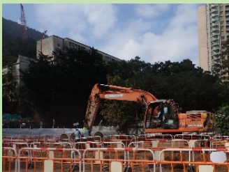
排水渠改道挖掘工程 Excavation Works for Drainage Diversion
