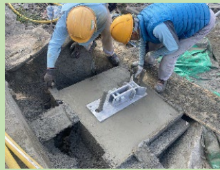
柔性防護網安裝工程 Installation of Flexible Barrier
