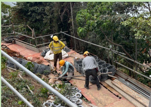
柔性防護網安裝工程 Installation of Flexible Barrier
