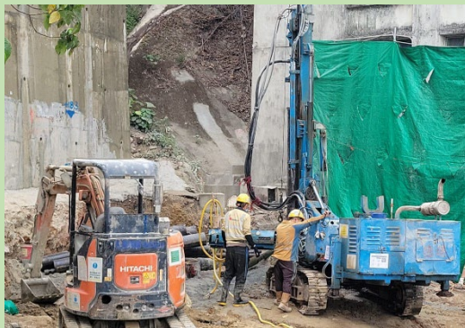
橋墩打樁工程 Piling Works for Bridge Pier Construction
